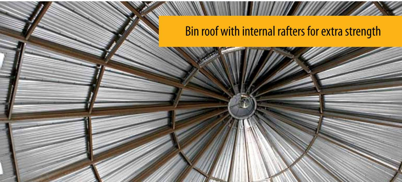
Bin roof with internal rafters for extra strength
